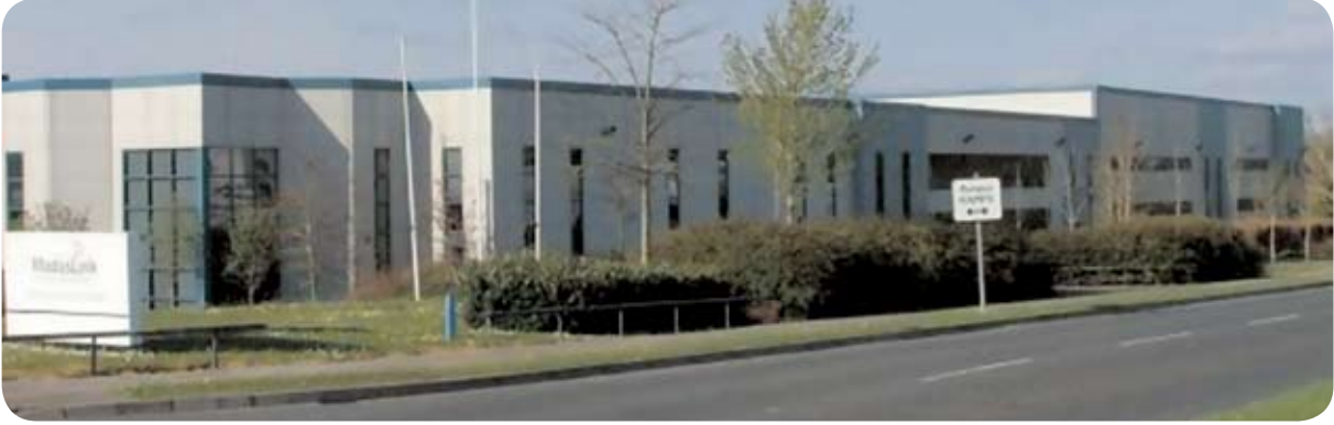
Green Data Centre
